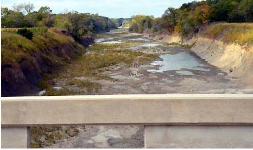
Erosion has transformed a relatively miniscule 16-feet wide, 10-feet deep channel that was excavated in 1928-29 into a 300-foot wide channel that continues to erode. *photo by Allen Rich*
